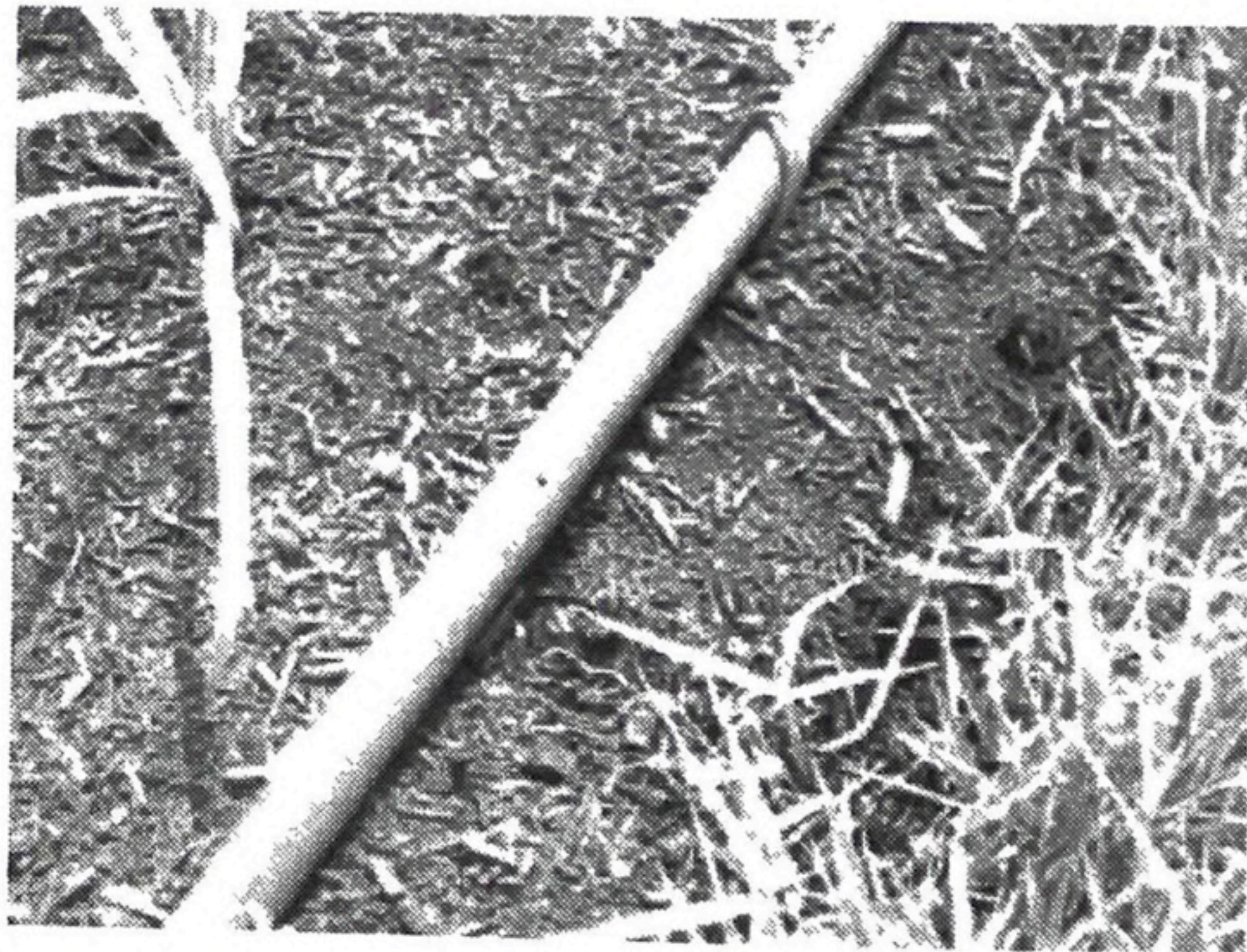
Photo 4-6 Pipe line for watering June in 2004
